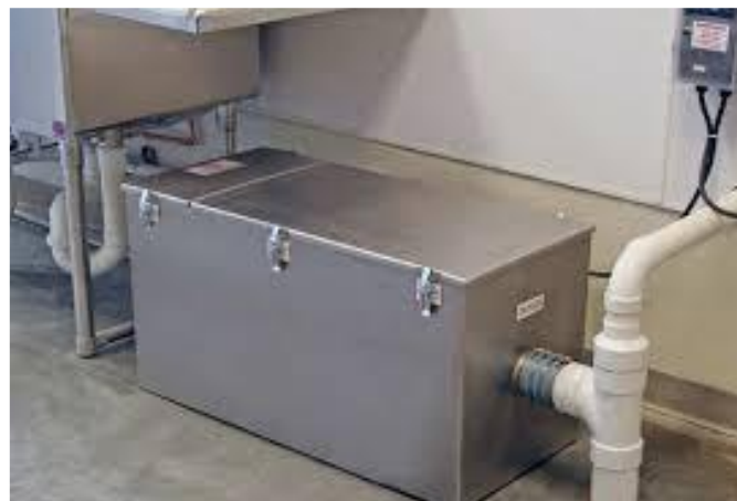
Gambar 8. Bak penangkap lemak ( grease trap )
